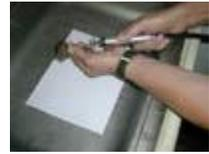
4. Trim the capillary tubing on the old gauge a couple of inches from the gauge head.
