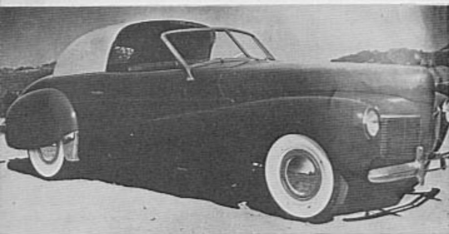
Another Coupé 66 Ville is shown here on a 1941 Mercury chassis. Note how the body has been lengthened for greater wheelbase by increasing the depth of the cowl section—between the dashboard and hood bonnet...
